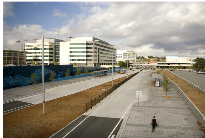
Recently upgraded Belconnen Bus Interchange
