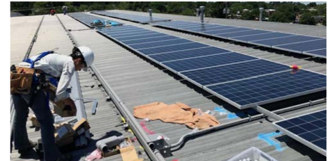
SOLAR PANEL INSTALLATION AND ROOFTOP WATER COLLECTION
