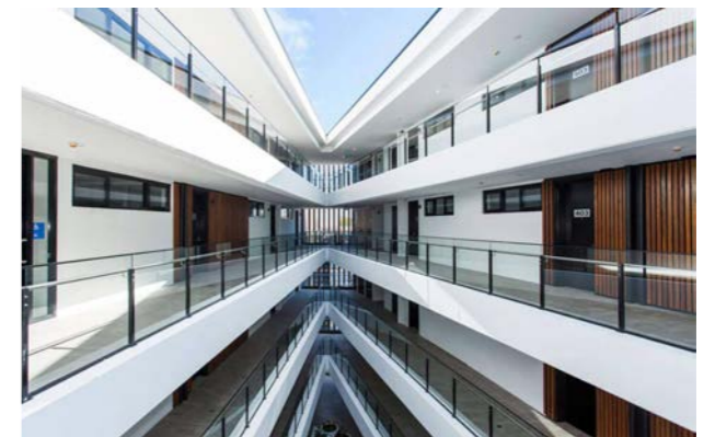
ATRIUM PROVIDING NATURAL LIGHT AND VENTILATION
